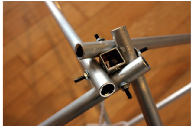
Fig. 8 Basic reciprocal structure, figure reprinted from [21]
